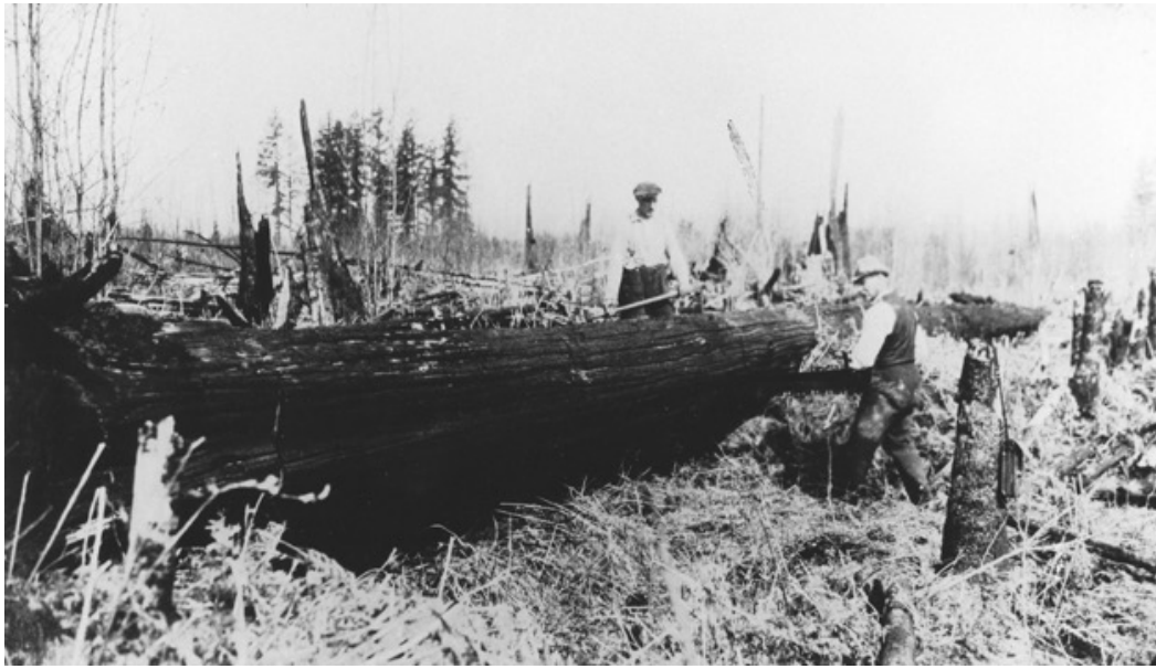
Clearing land on Langley Prairie, c. 1920. Langley Centennial Museum Photo #1306
